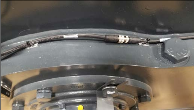
Figure 38 – Sensor cables secured with cable tie mounts
